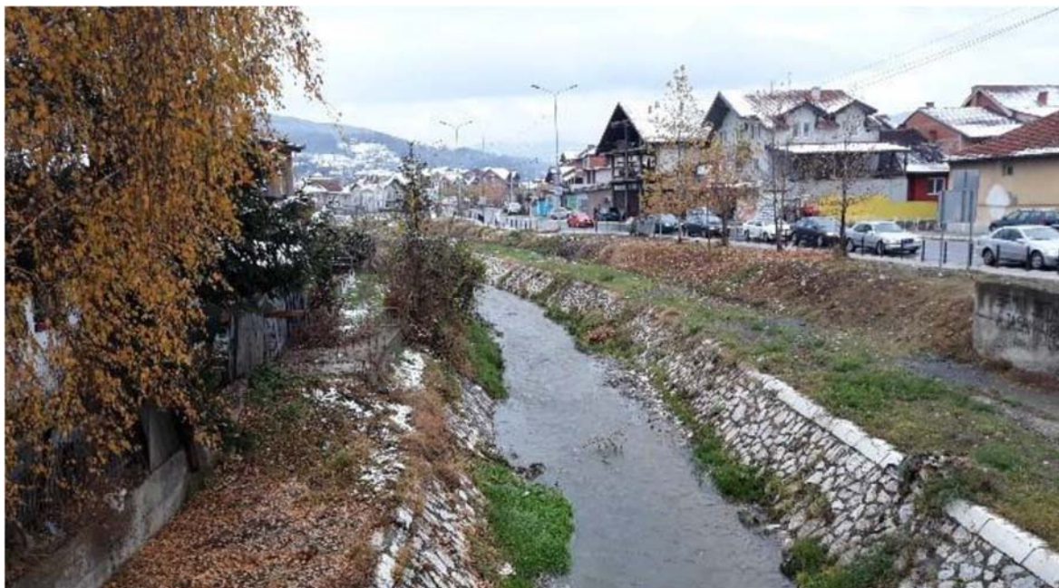
Figure 4 Trained section of Jovanica River through the city of Novi Pazar
